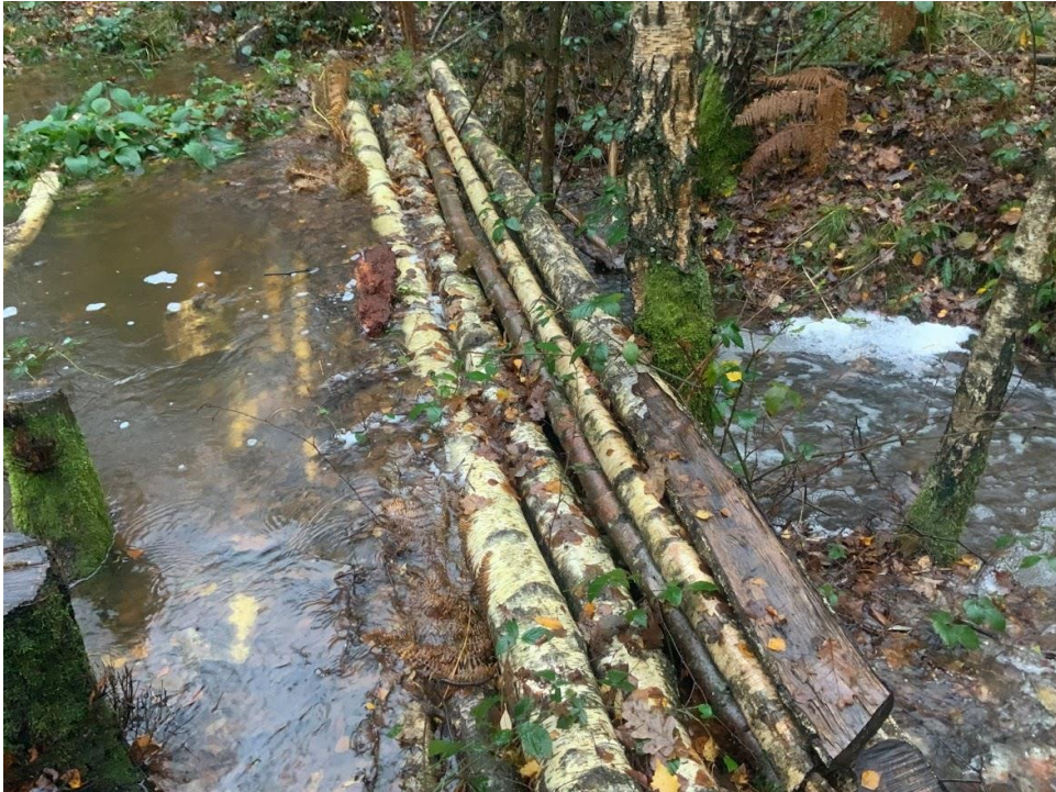
Leaky dam in action
