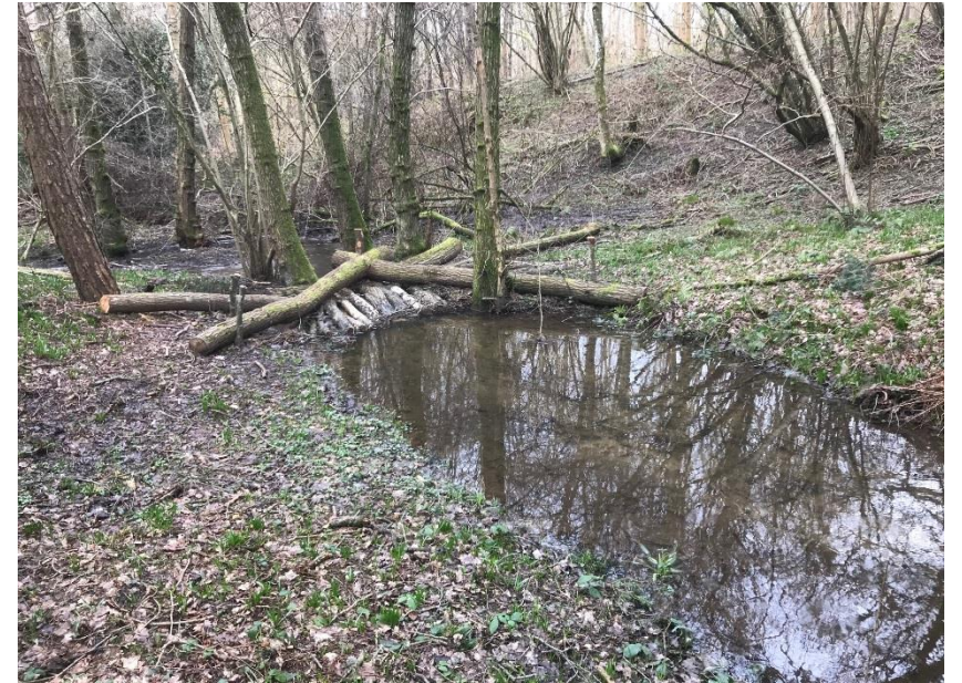
Leaky wood structure Alder Stream
